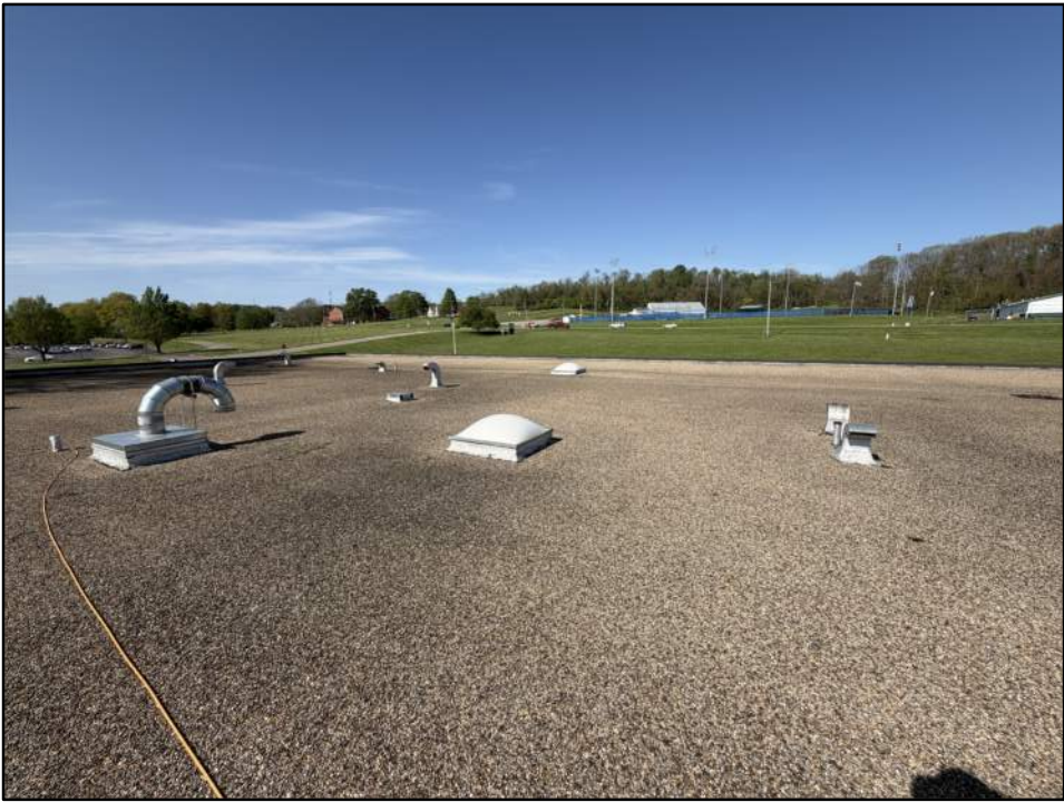
GENERAL ROOF PICTURE SHOWING SKYLIGHT AND INTAKE DUCTWORK
