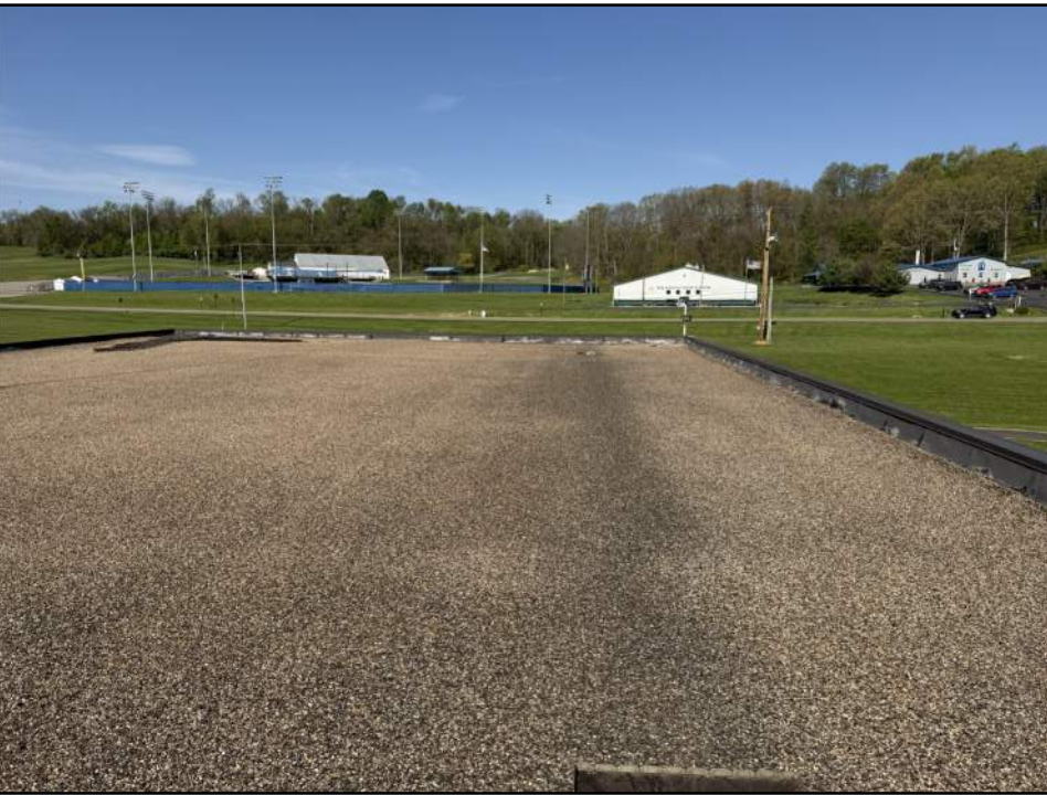
GENERAL ROOF PICTURE
