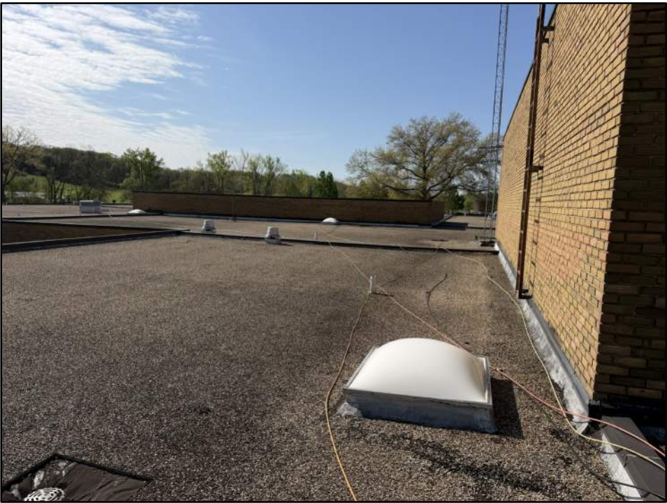
GENERAL ROOF PICTURE W/ SKYLIGHT
