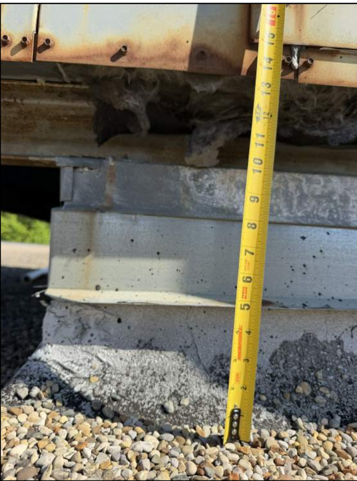
EXISTING RTU CURB HEIGHT
