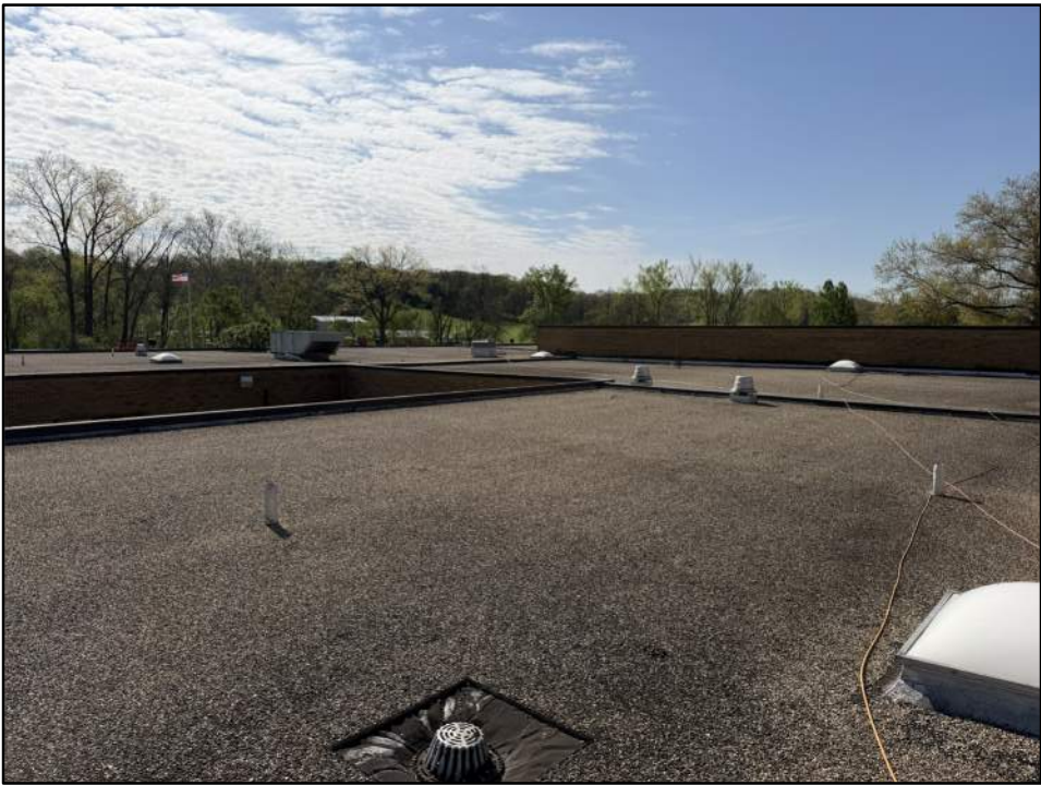
GENERAL ROOF PICTURE
