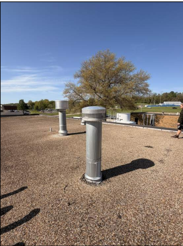
EXISTING BOILER FLUES TO REMAIN
