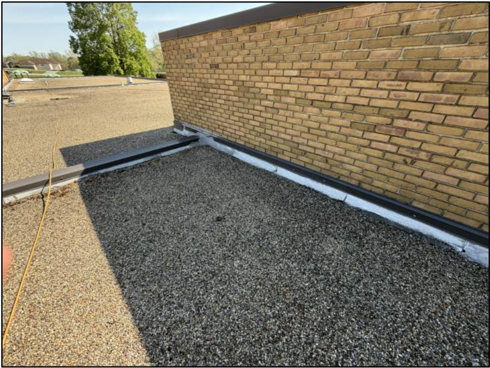
ROOF PICTURE SHOWING EXP JOINT AND WALL FLASHING
