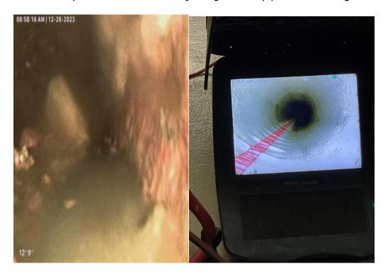
The photos below are images of the broken access drop in the SSA area and the same area as the sanitation line was being relined.
